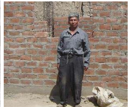
Another earthquake relief house going up in Pisco.
